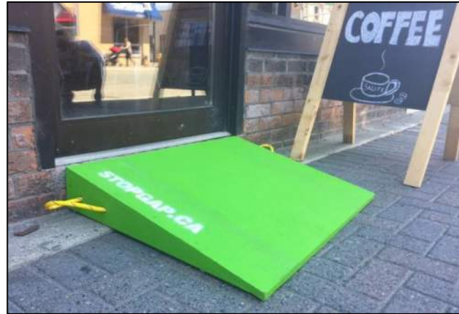
Customized portable ramps are a simple method / interim measure to improve accessibility (Image source: CBC News, Sudbury, July 5, 2017)
