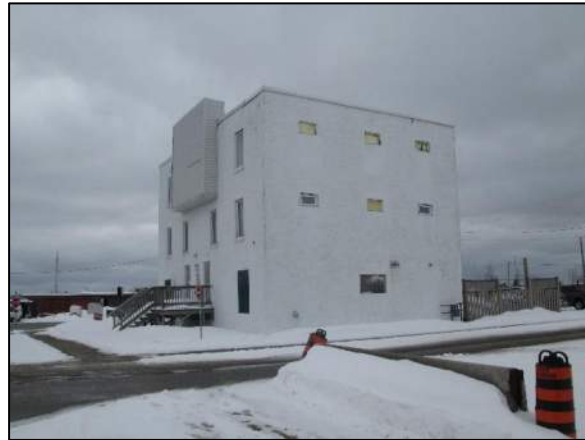
Image 16 – Vacant building with redevelopment potential in downtown
