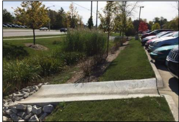
Example of a bioswale feature (Image source: Aaron Volkening, Flickr)
