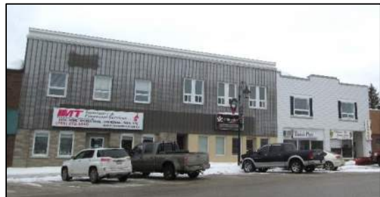
Existing upper storey residential units, Cochrane (Image source: WSP, 2018)
